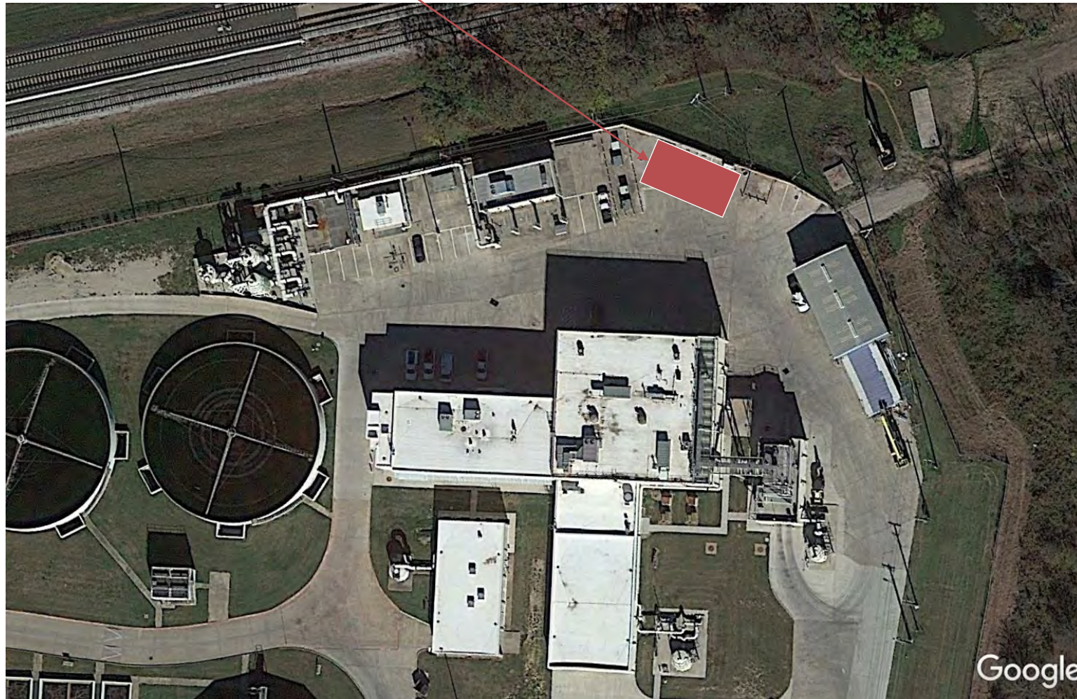
Rowlett Creek WWTP Transfer Pump Station
