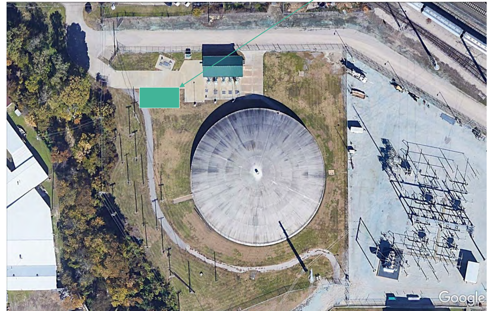
Lavon Pump Station
