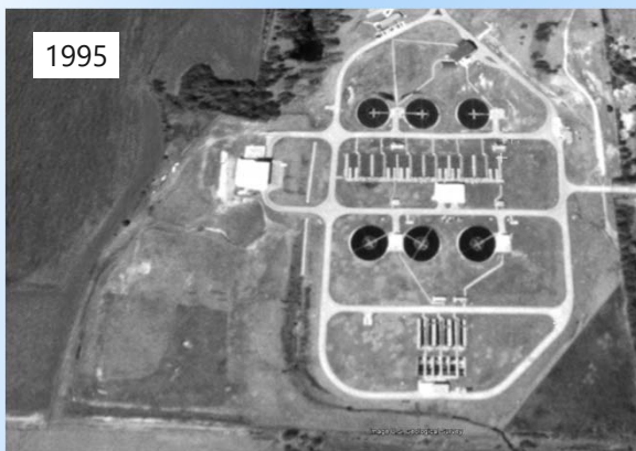
– Phase 1 construction in 1987
