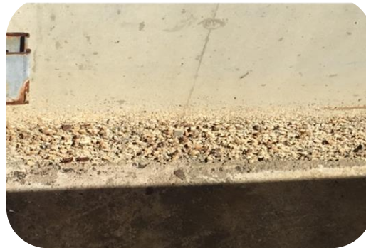
Cover any exposed aggregate/steel
