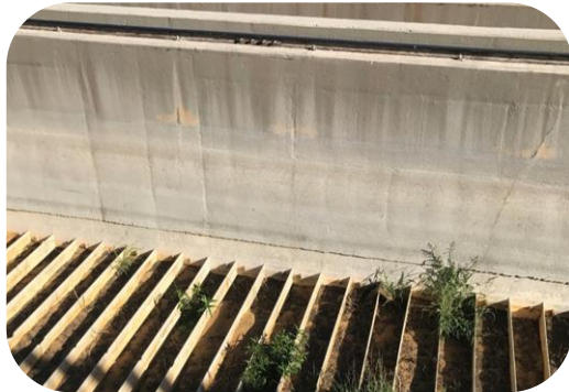
Repair major cracks
