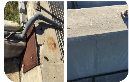
Repair minor cracks
