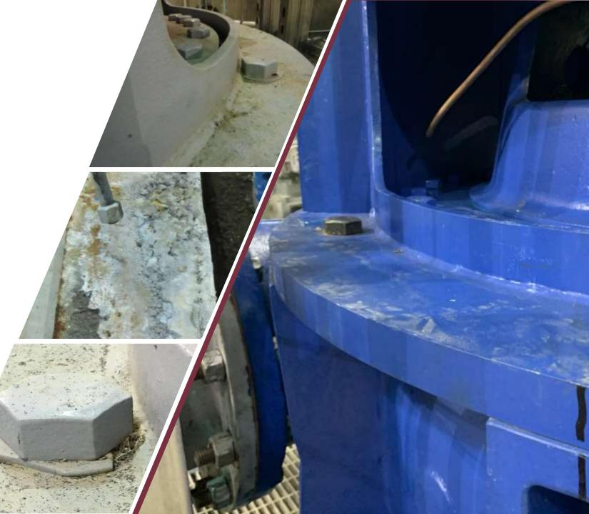
Inadequate pipe support results in nozzle loading
