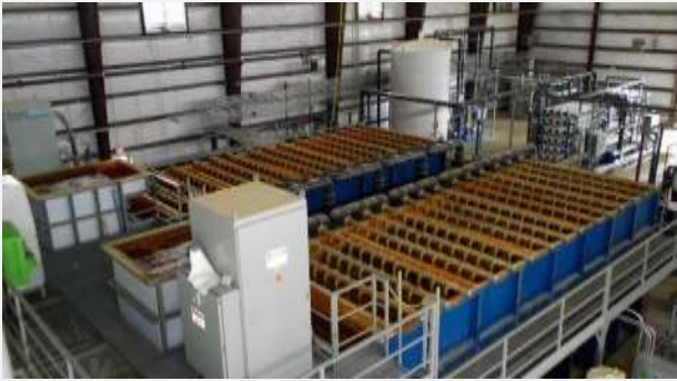
1,000 gpm Powell Water EC (left) followed by UF (right)
