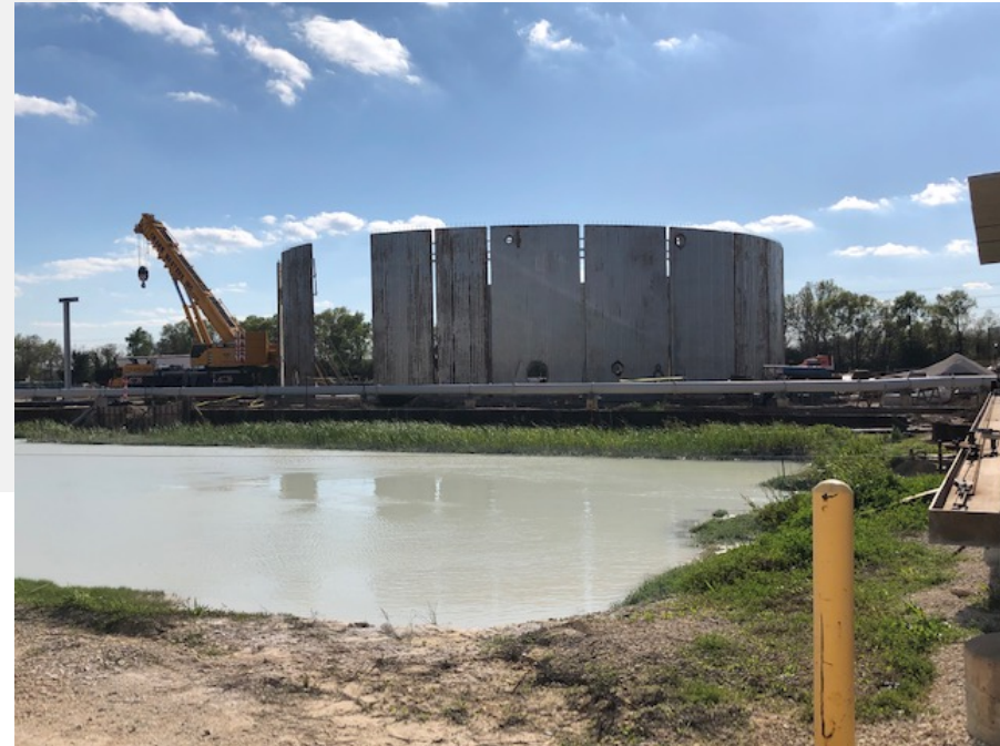
Drilling 197 Piers and Erecting Panels
