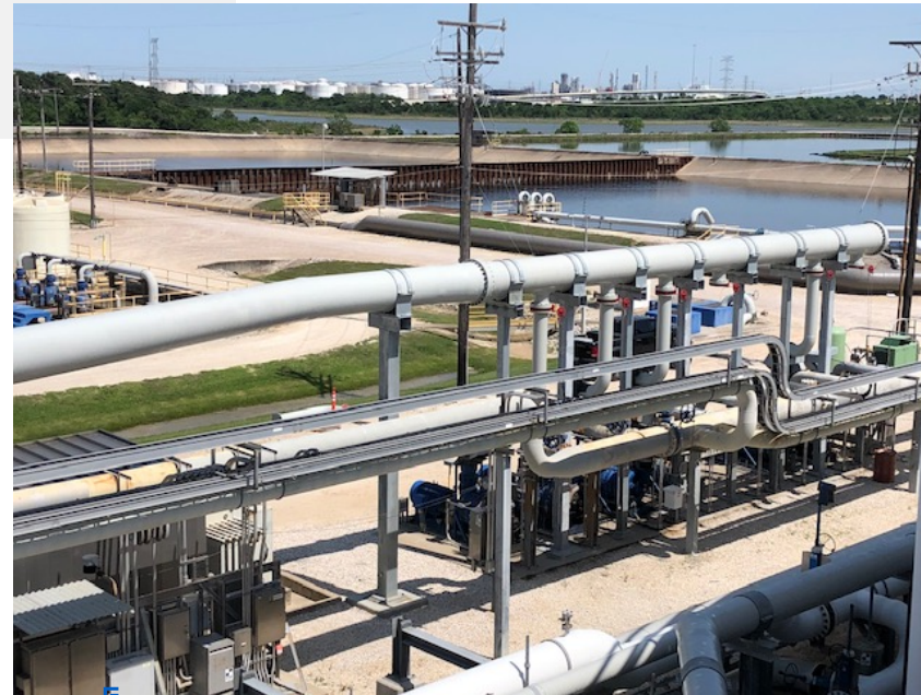
Piers, Supports and Piping Installed
