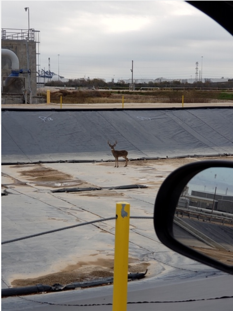
Buck Inside Newly Lined Pond 4
